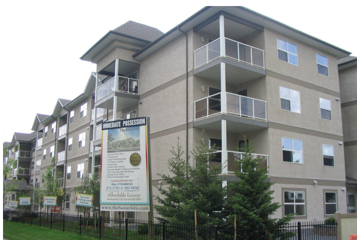
This private developer is selling new luxury condo apartments in Edm. for $85,000. Even lower costs are possible with economy of scale building and by reducing barriers that inhibit development of rental units.
